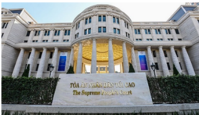
THE SUPREME PEOPLE'S COURT - VINHOMES HA NOI CITY Scope of supply: Condair dehumidifier
