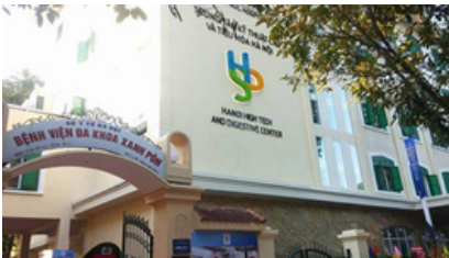
XANH PON HOSPITAL HA NOI CITY Scope of supply: HVAC Control system
