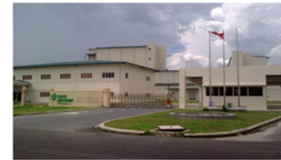
OLAM ALMOND BIEN HOA FACTORY DONG NAI PROVINCE Scope of supply: Sensible heat recovery wheel Seibu Giken For production area
