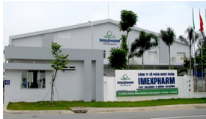
IMEXPHARM PHARMACEUTICAL FACTORY HO CHI MINH CITY Scope of supply: Sensible heat recovery wheel Seibu Giken For production area
