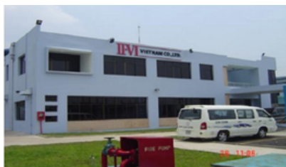
II-VI VIETNAM FACTORY BINH DUONG PROVINCE Scope of supply: Air-cooled mini chiller TICA For production area
