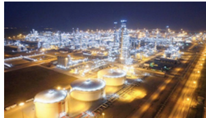
NGHI SON OIL REFINERY PLANT THANH HOA PROVINCE Scope of supply: Condair humidifier For production area
