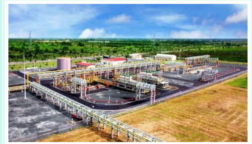
CA MAU GAS PROCESSING PLANT CA MAU PROVINCE
